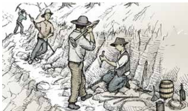
Construction workers preparing rock for blasting on the ditch (A Swift)
